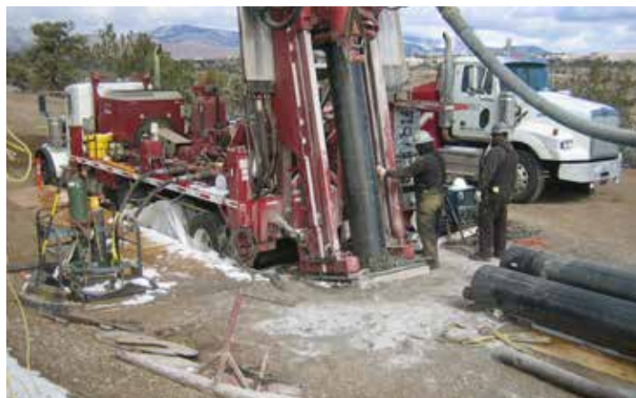
Angle drilling of remediation well
