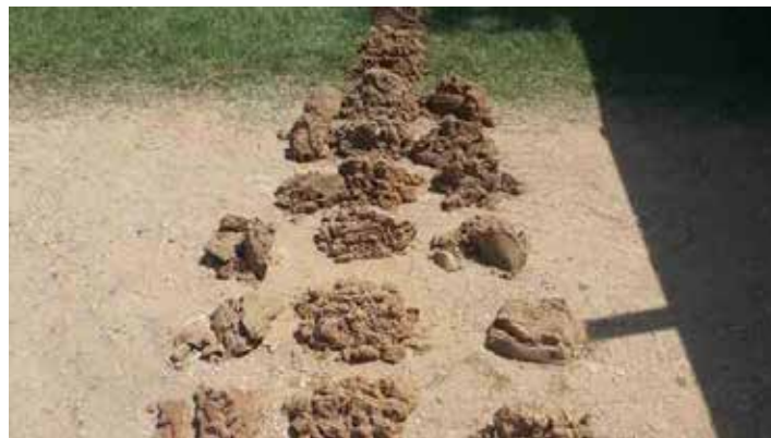
Cuttings at a jobsite where a wellfield was being expanded for the city of Cunningham, Kansas. Photo courtesy Ned Marks, Terrane Resources Co.
